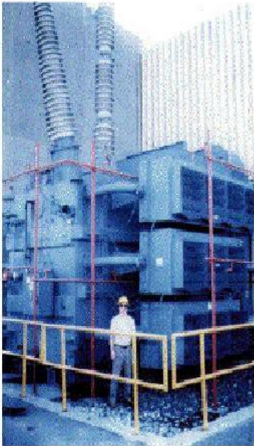
A large space storm in 1989 caused currents which damaged this transformer and shut off power for six million people for nine hours.
